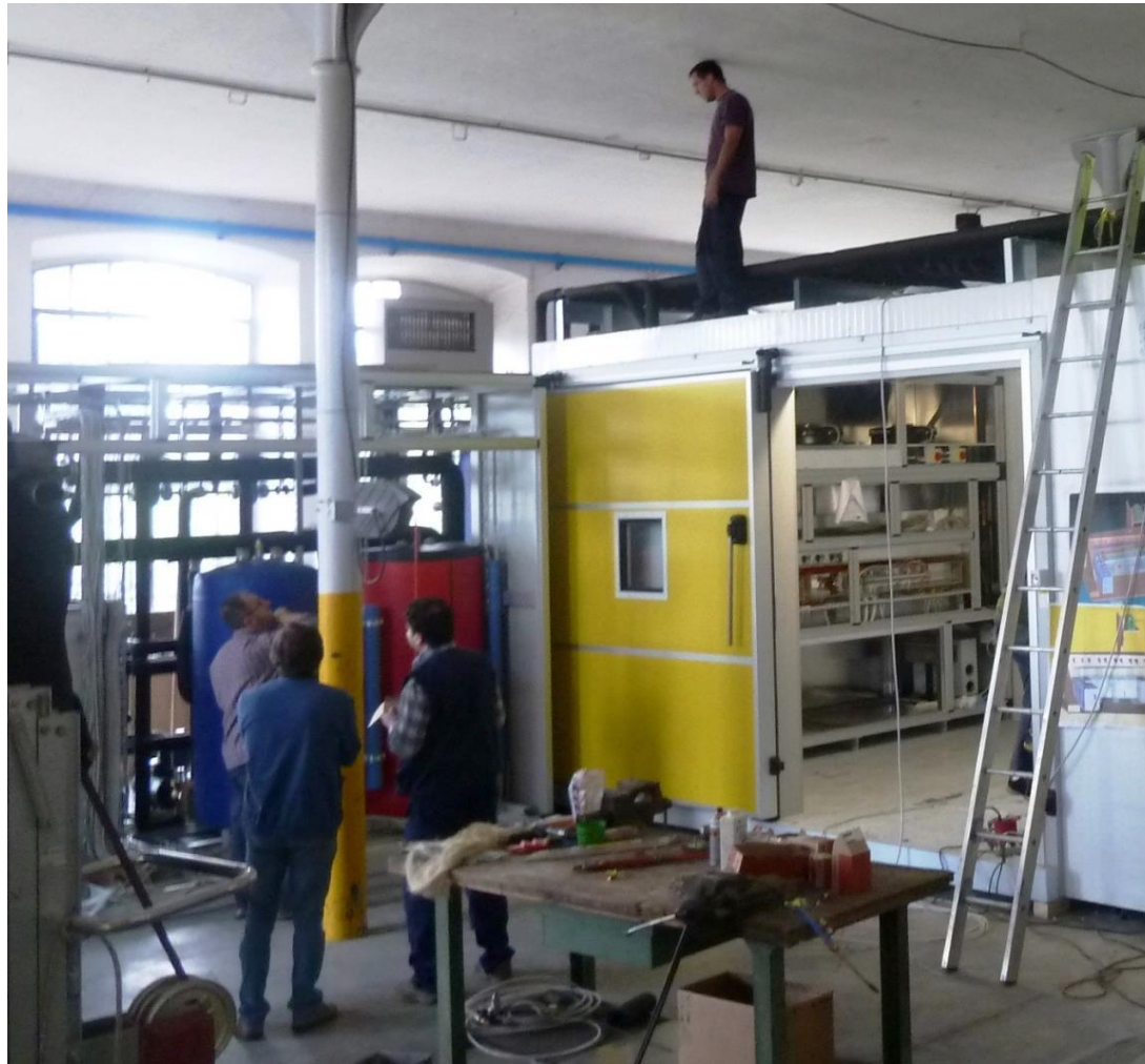
Climate chamber under construction
